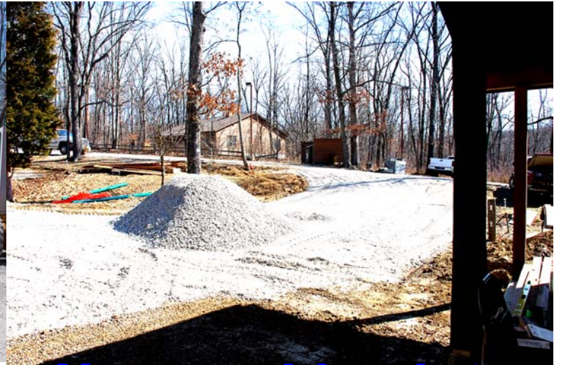
New parking lot (in progress)
