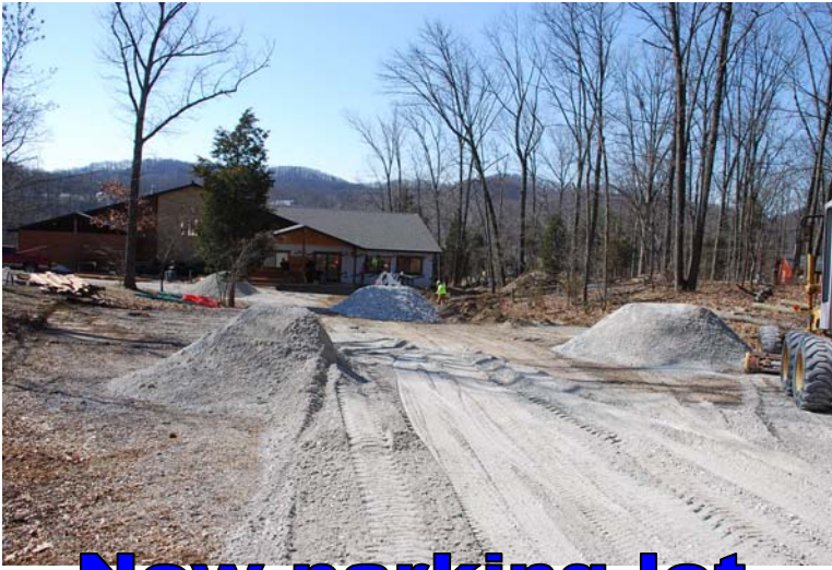
New parking lot (in progress)
